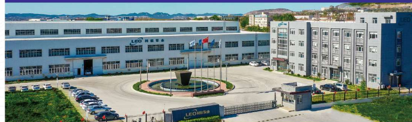
Pump Manufacturing Base for Petrochemical Industry
